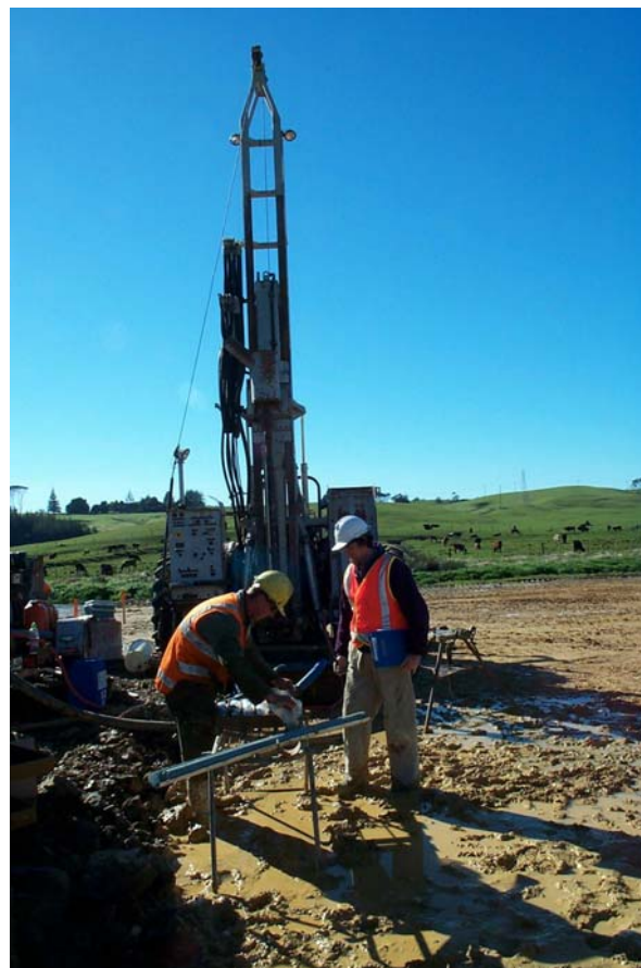
Figure 4. Installing Inclinometer / Sondex System
