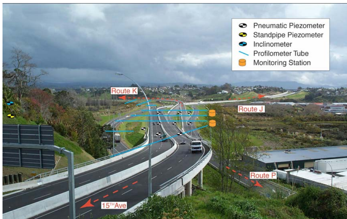
Figure 11. The completed PJK Interchange, showing instrumentation lines and monitoring locations.
