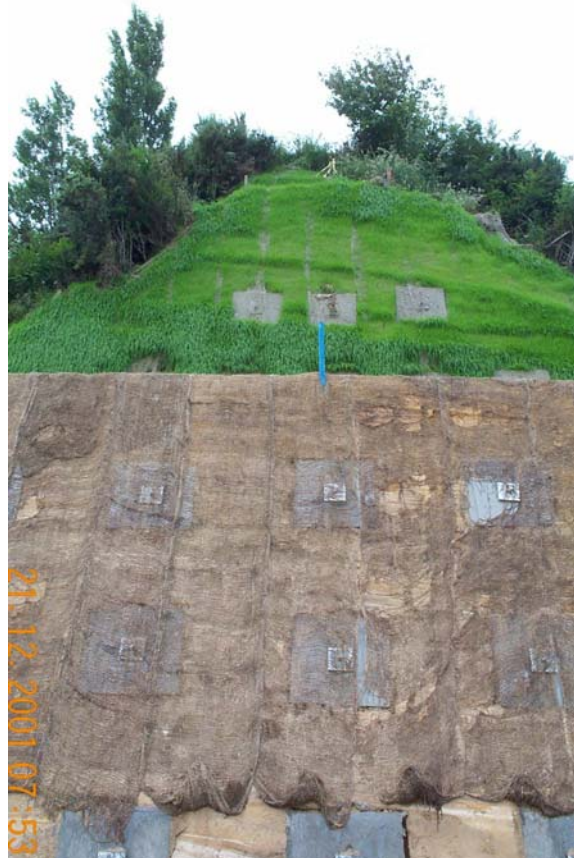
Figure 15. Soil Nailing / Inclinometer Installation. PJK. (K6 Cut)
