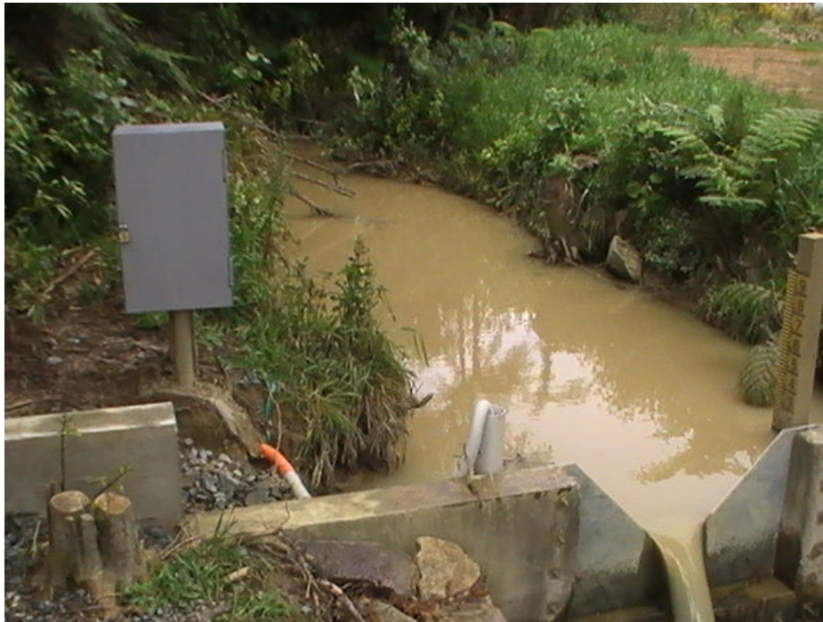
Figure 1-Weatherproof enclosure and weir at Site 2, Tip Stream, below Silverstream Landfill settlement pond.
