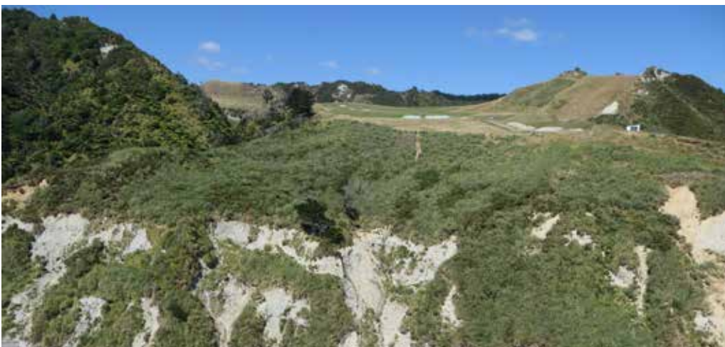
Looking upslope. Gently sloping grassed area on top with active landslide area visible in the center of the photo.
