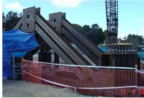
Figure 4: Test pile reaction frame
