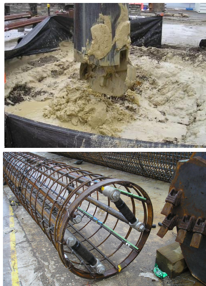
Figure 2b: Pile spoil grouting pipe work
